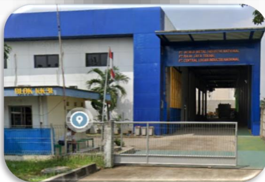
Fabrication Workshop JABABEKA Industrial Park II
