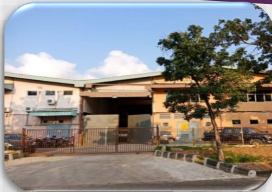
Head Office & Fabrication Workshop JABABEKA Industrial Park I
